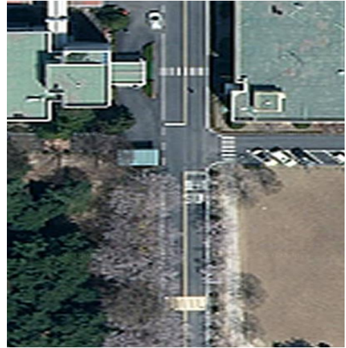
Figure 12. Well-structured noraml road which has lanes and curbs
